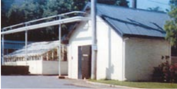
Boiler room and hot house
