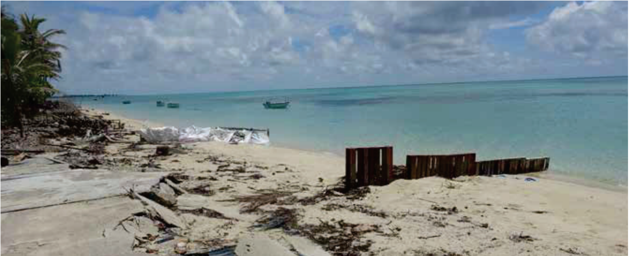
Makeshift groynes made from pallets and destruction of property by high tides, Masig Island. Credit: Sophie Marjanac, ClientEarth
